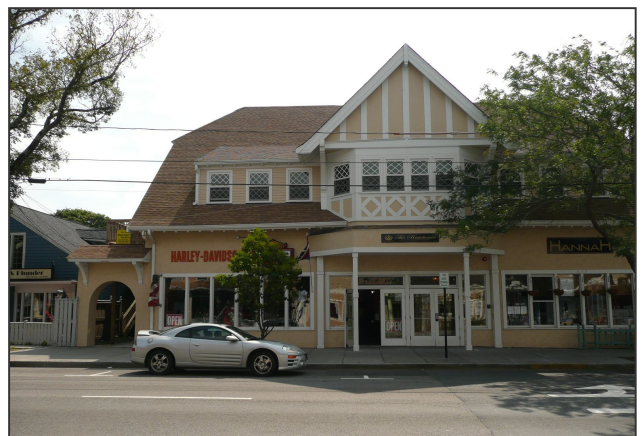
The historic Hyannis Theatre was renovated into a mixed-use residential and retail building.
