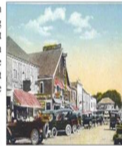
Historic building spacing on the east end of Main Street.
