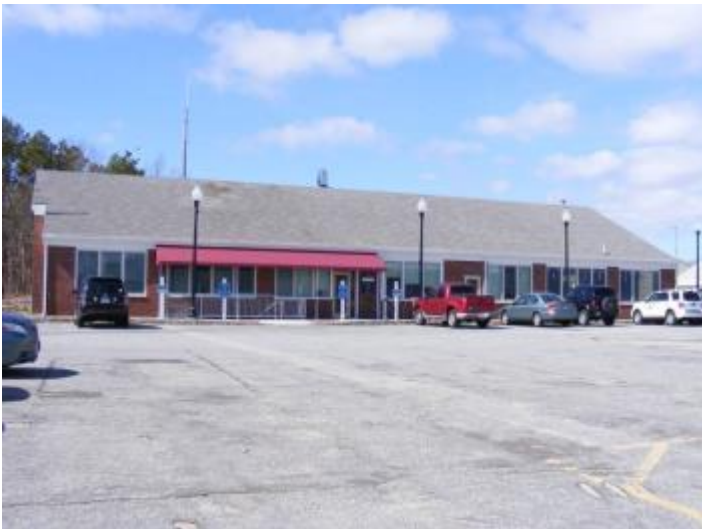
Department of Public Works Offices
