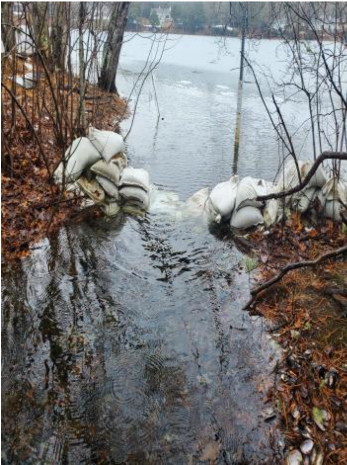
Long Pond Centerville Outlet (facing the pond). Taken January 2021
