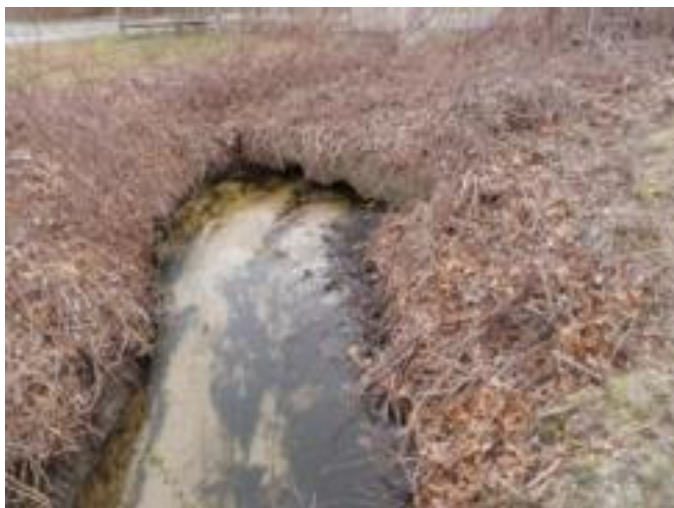
Culvert under Lake Elizabeth Drive (Restriction 1)
