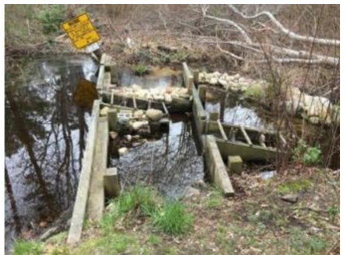
Fish Ladder/Dam at Lake Elizabeth (Restriction 2)
