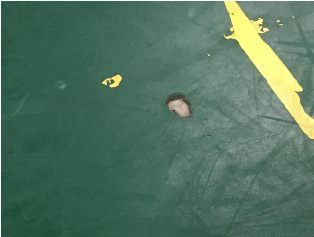
GYM and Field House Floor
