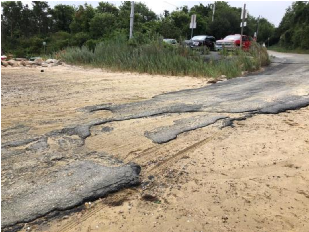
Scudder's Lane Boat Ramp
