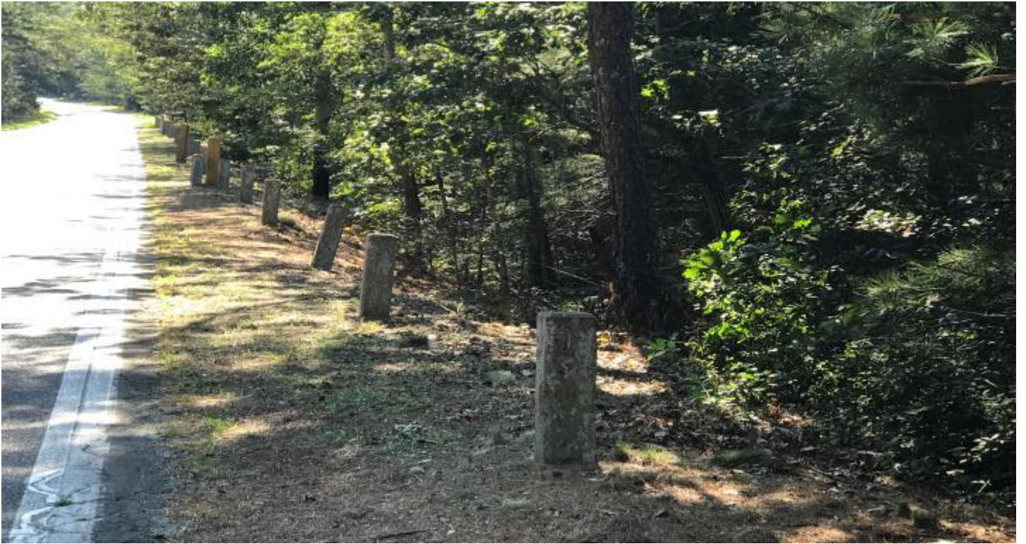
Concrete Guardrail Removal
