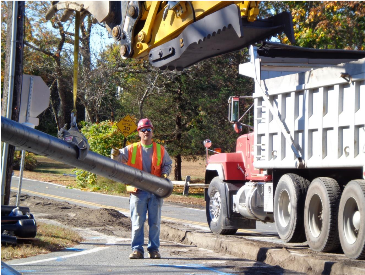
Pipe Replacement Project
