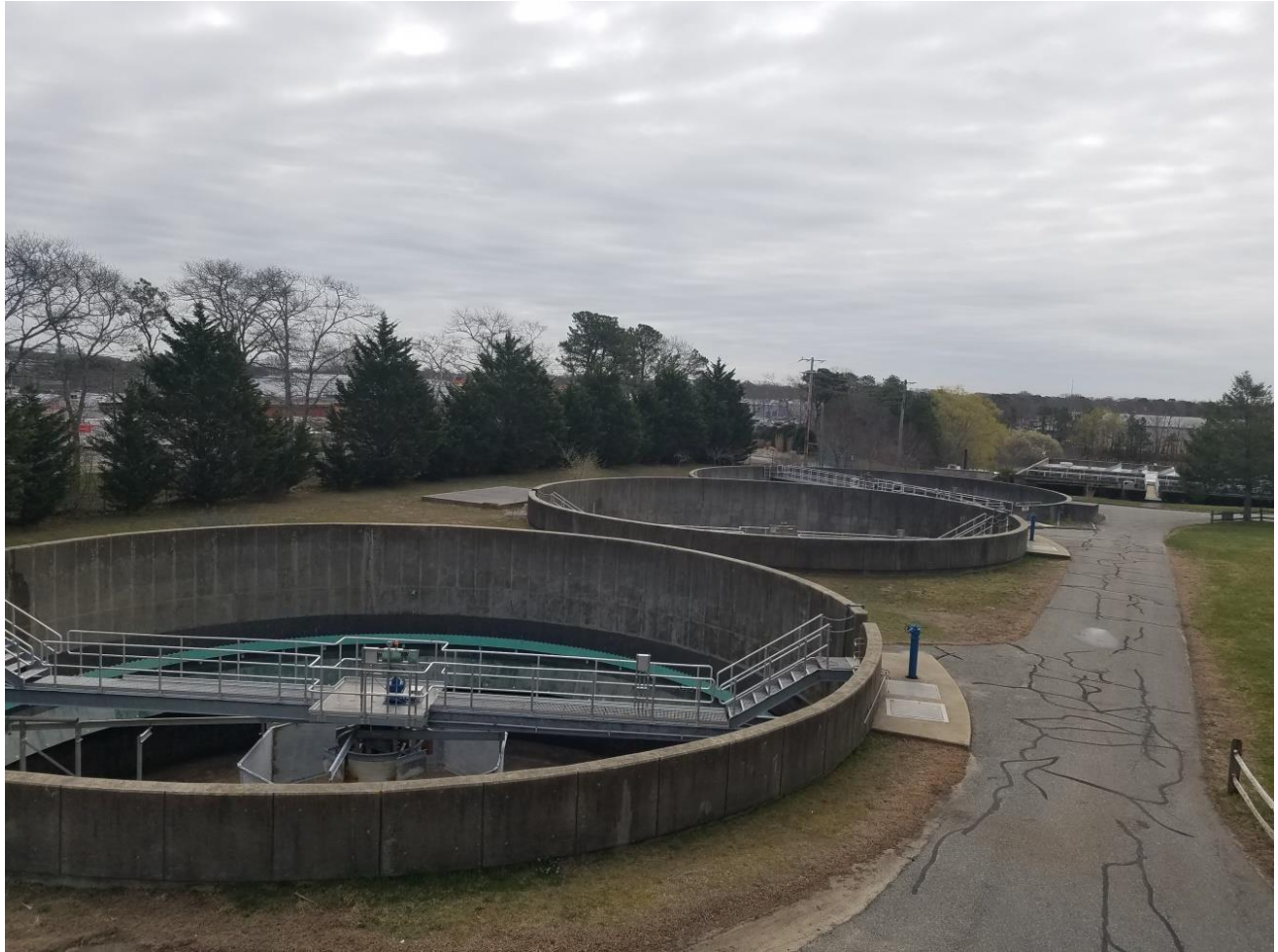
Clarifiers at the Wastewater Pollution Control Facility
