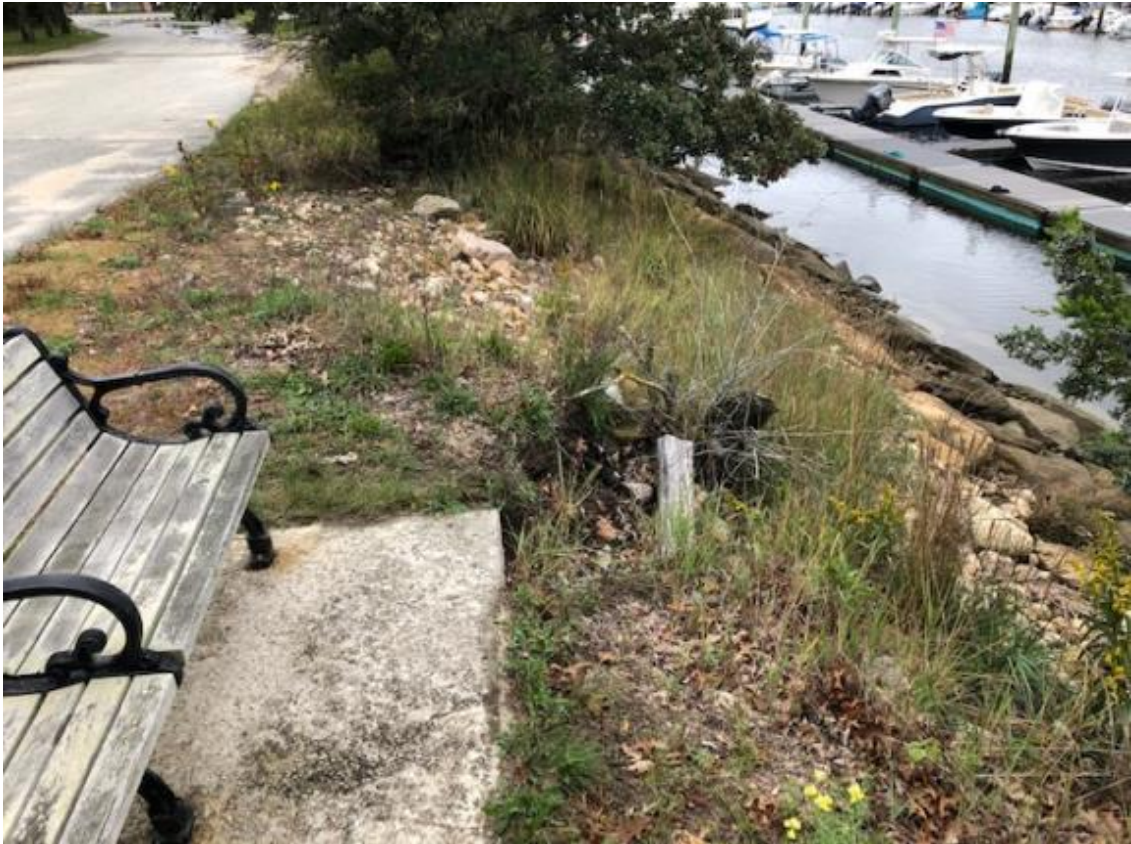
Barnstable Harbor Marina Revetment
