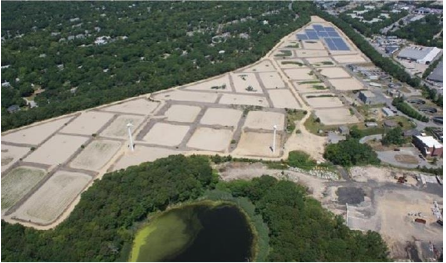
Wastewater Treatment Facility Effluent Disposal Sand Beds
