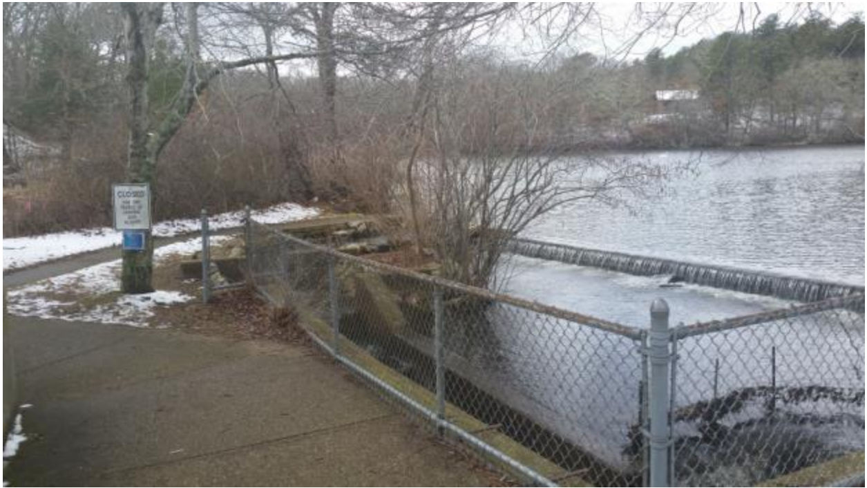
Mill Pond Dam and Fish Ladder
