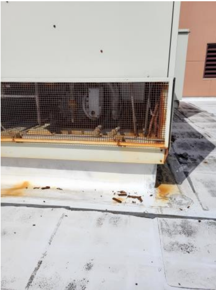
Roof Top Unit Ventilators
