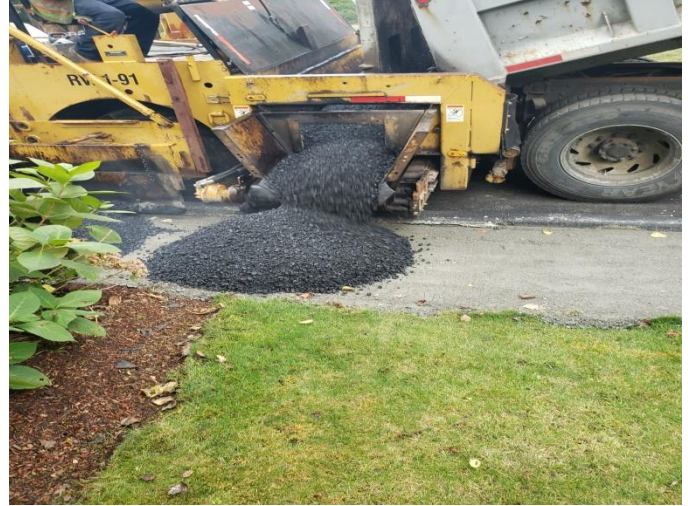
Glen Eagle Drive Road Project
