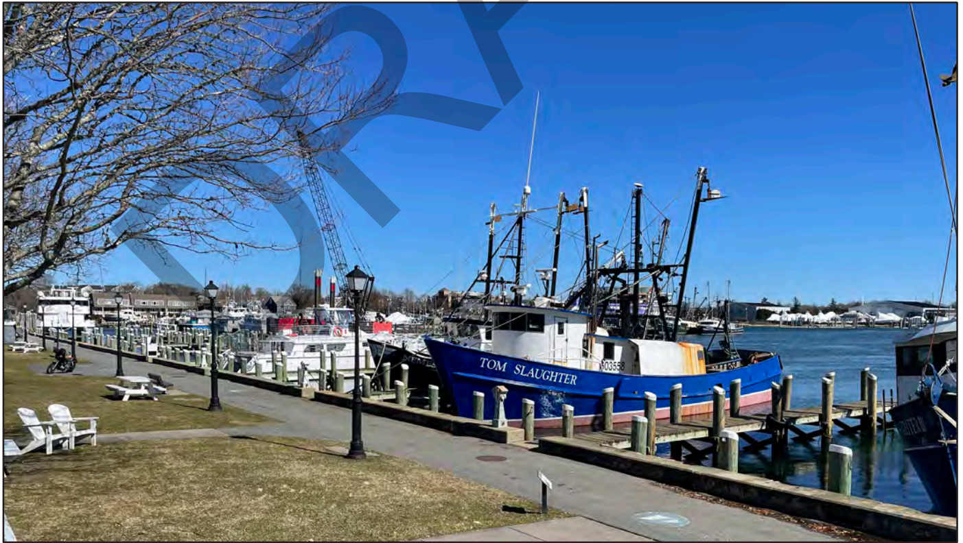
Figure 5 Photograph 2: View of the Harborwalk in Bismore Park looking northeast Source: Tetra Tech, 2024
