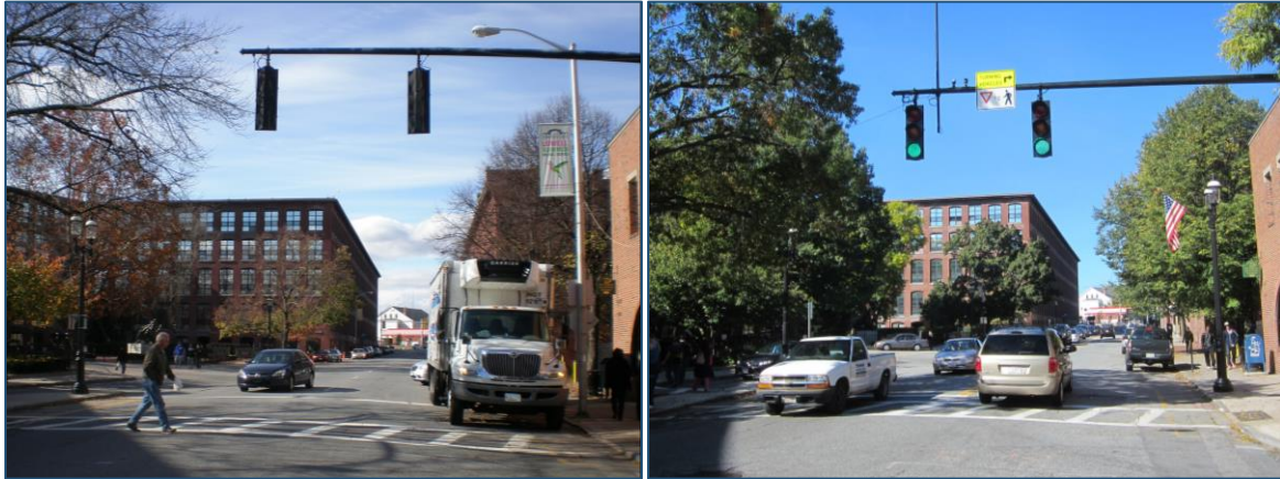
Figure 15 Market Street Before and After
