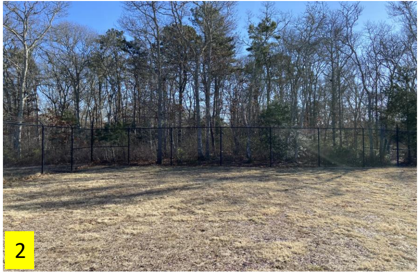
View south towards future new Straightway Facility area
