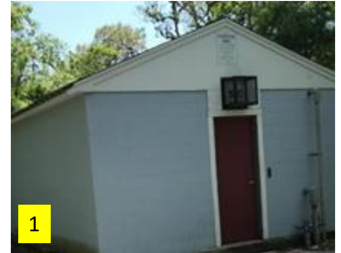
Existing Simmons Pond Pump Station
