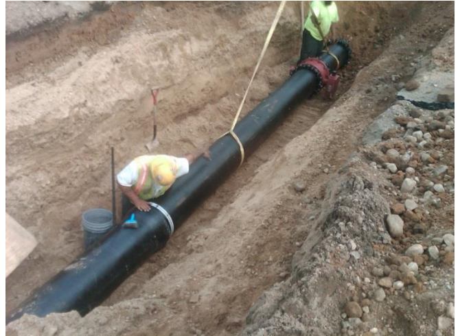
Pipe Replacement Project
