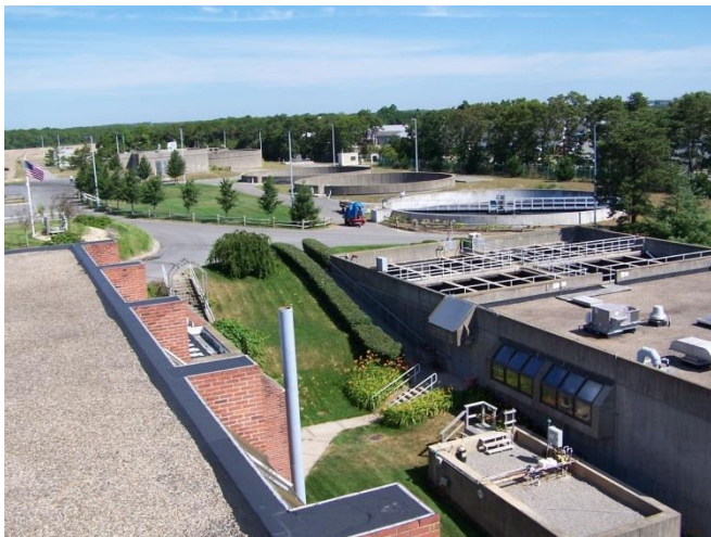
Waste Water Facility
