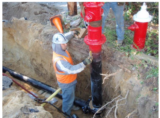
Public Fire Hydrant Installation
