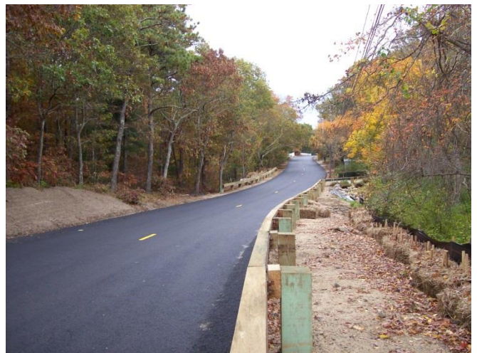
Completed Road Pavement and Guardrail
