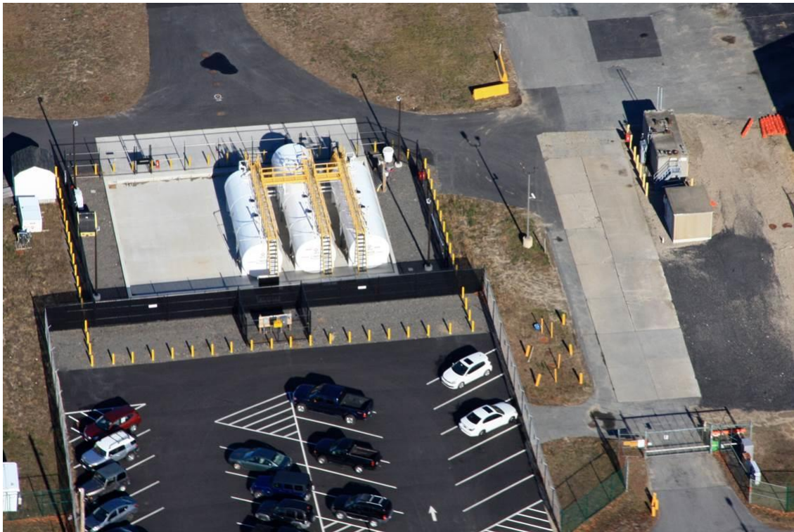
February 2017 Aerial of the New 60,000 Gallon Above Ground Jet Fuel Storage Tanks And New Employee Parking Lot Leased by Cape Air
