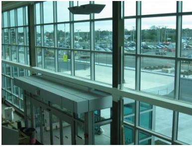
Inside Main Terminal
