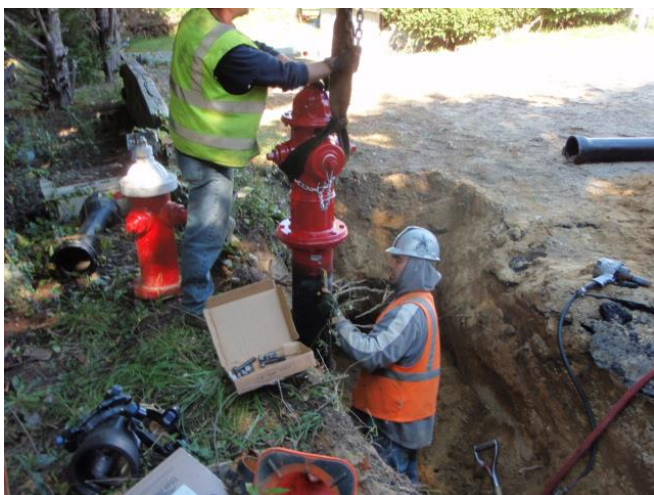
Public Fire Hydrant Installation
