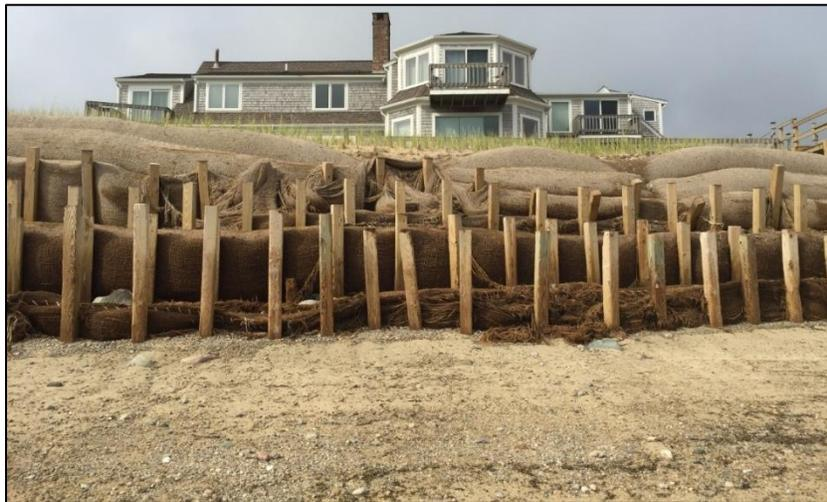
**Figure 16. Example of failed sand-filled coir bag system.**
